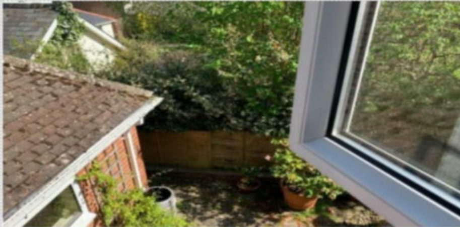
Fig. 3: View from upstairs towards the rear elevation of the Applicant's garage (top left of the image). The proposed extension sits only ~300mm lower than the ridge of the existing garage.
